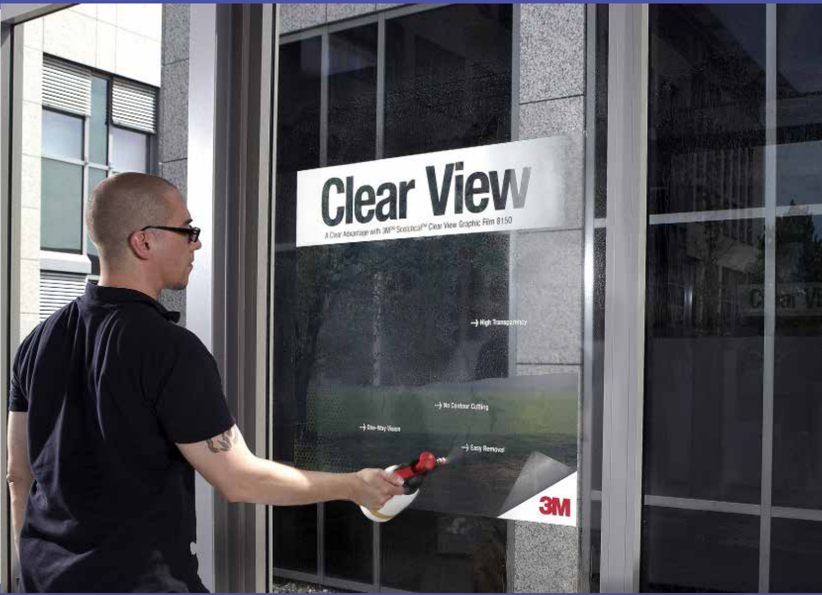
Making a perfect wet application of 3M™ Scotchcal™ Clear View Graphic Film 8150 | Step 18:
